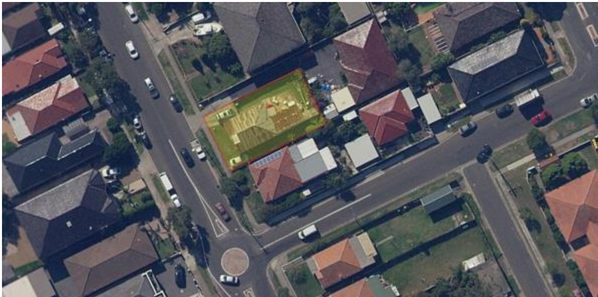
Subject Site: 98 Moreton Street Lakemba
