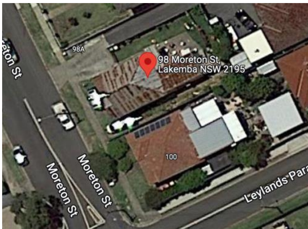
Existing front setbacks at 98 and 100 Moreton Street
